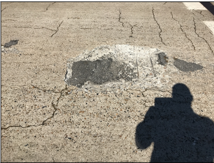
Span 1 large spall with exposed rebar at centerline
