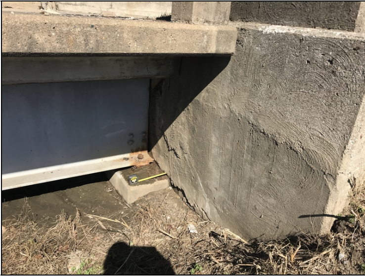
Bent 4 abutment the back wall is sheared and leaning against bridge deck closing deck joint.
