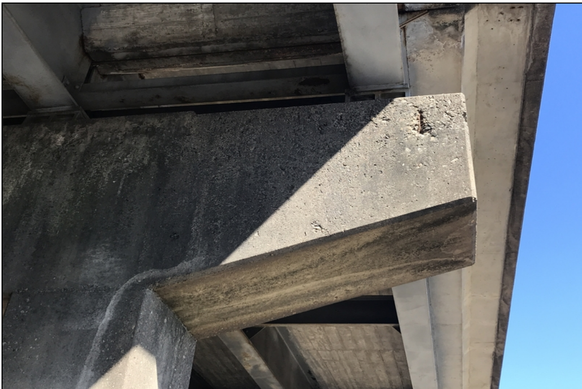
Bent 3 cap spall with exposed rebar
