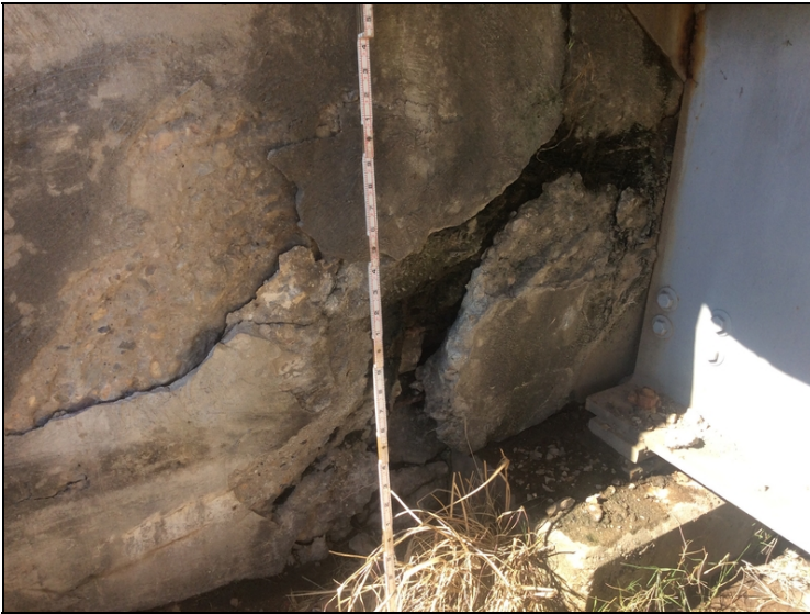
Bent 1 abutment the back walls are sheared and leaning against bridge deck closing all deck joints and causing hard impact to span 1.
