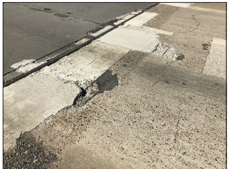
Large spalls with exposed rebar and spalls filled with asphalt in span 1.
