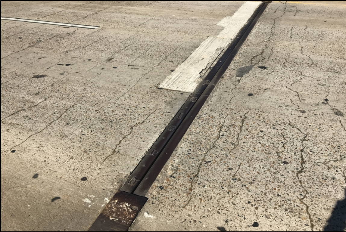
Span 3 deck plate is missing
