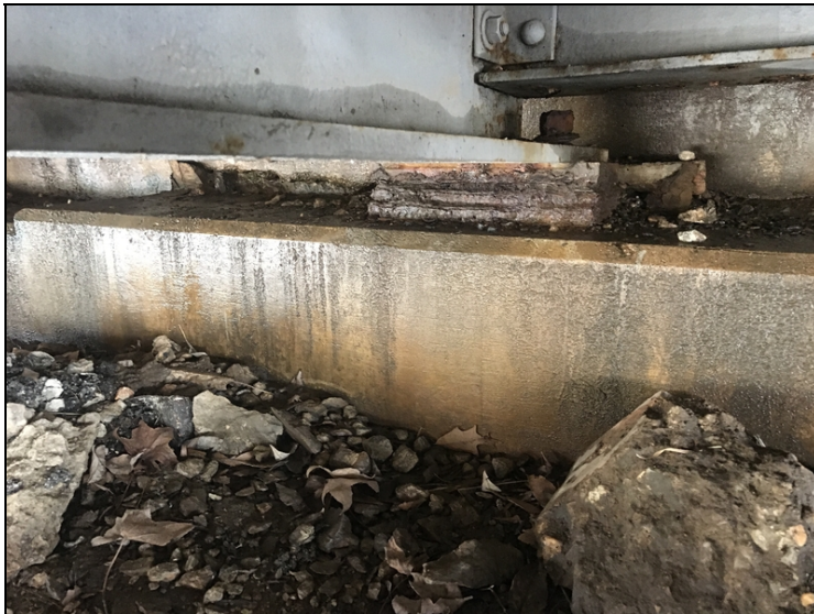
Bent 1, girder 2: bearing has active corrosion with section loss to it. This is condition is similar to the other bearings at this bent.
