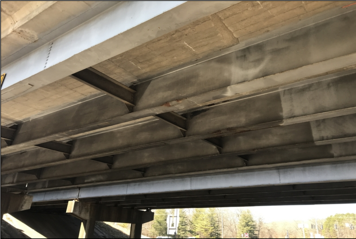
Span 2 minor damage to beams from traffic impact
