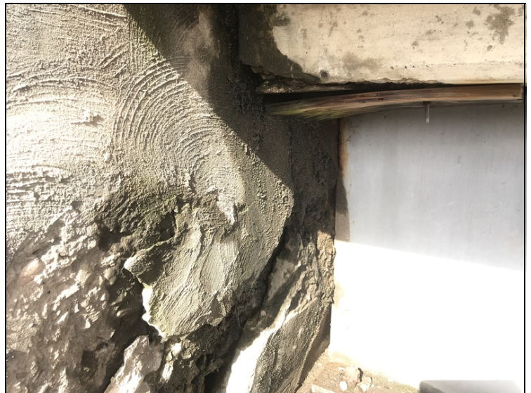
Bent 1: the back wall is broke and is leaning against the girders. The back wall has spalled in numerous places and exposing rebar
