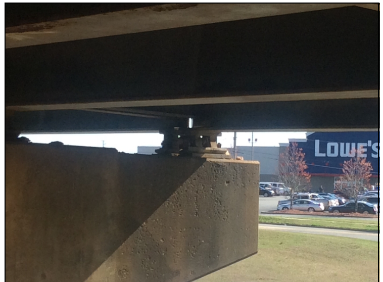
Bent 2 beam 5 bearing is fully rotated
