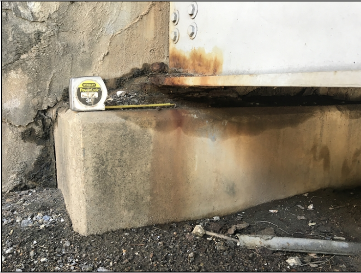
Bent 1 bearing 1 corrosion
