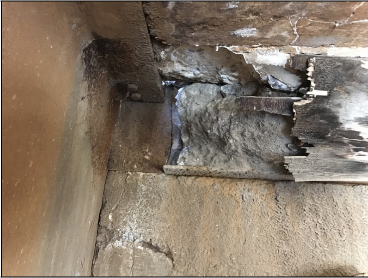
Span 1 Previous patch is failing. Daylight can be seen through patch.
