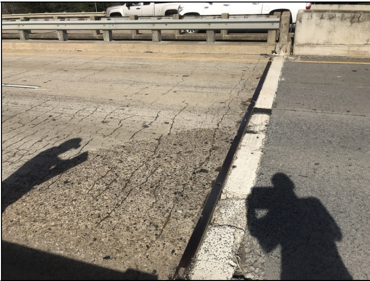
Bent 4: joint material is missing and the joint has completely closed. Similar condition is at bent 1 and 3.
