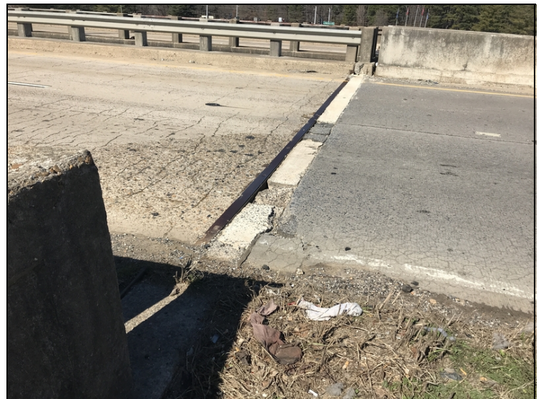
Bent 4 top of back wall has large spalls and spalls filled with asphalt
