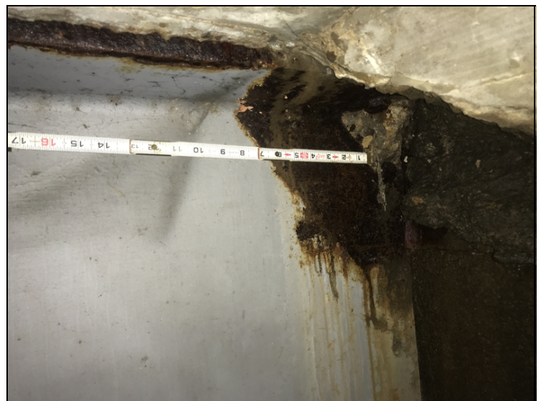
Span 1, girder 2: the haunch has pitting
