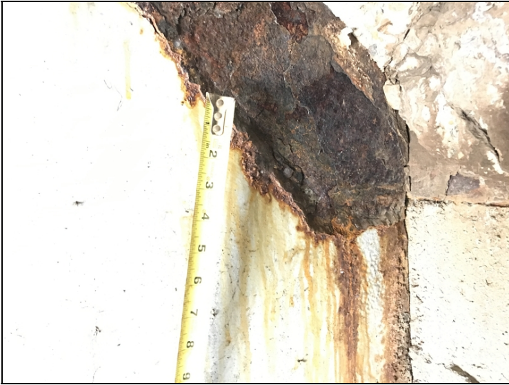
Span 3 Beam 3 at bent 4 has a 1" hole in web and active corrosion to haunch.
